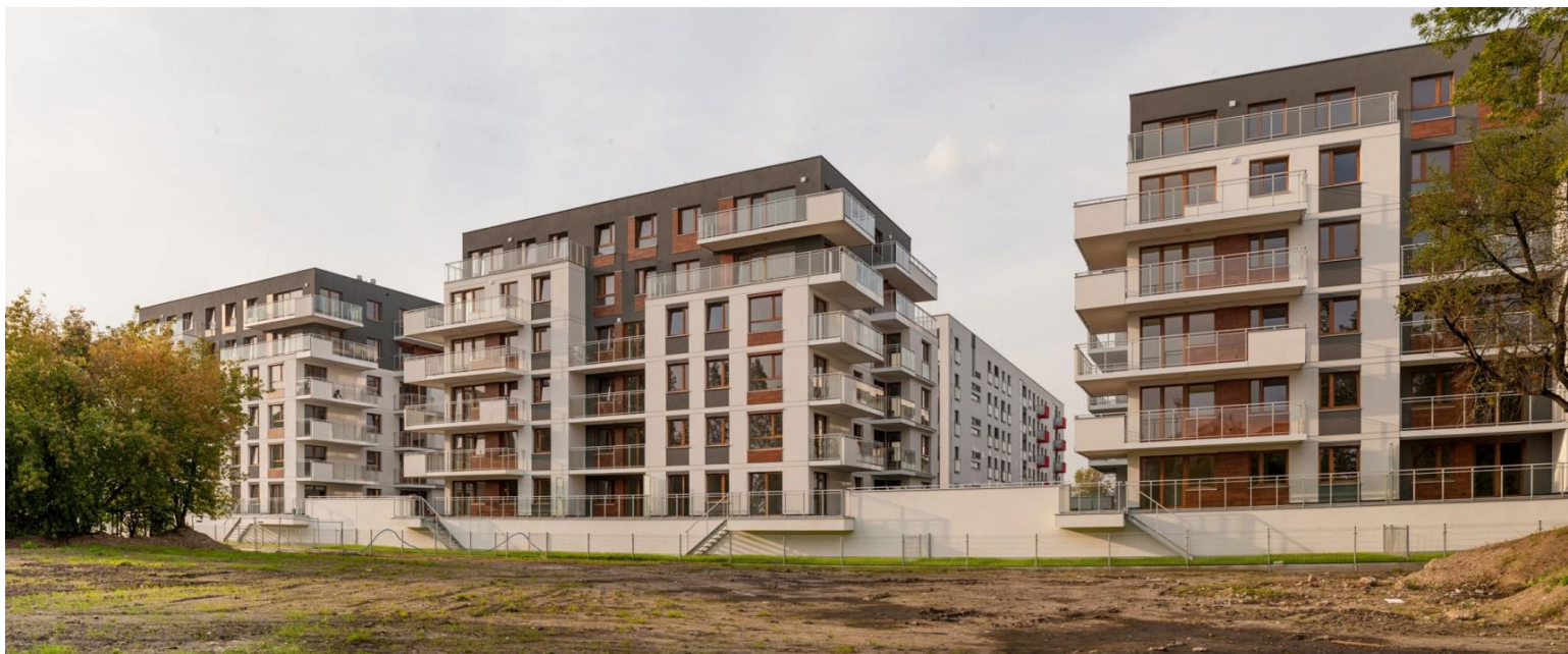
Stages VI & VII, OSIEDLE-INNOVA, 531 apartments and 4 commercial premises., Wrocław (September 2014).
